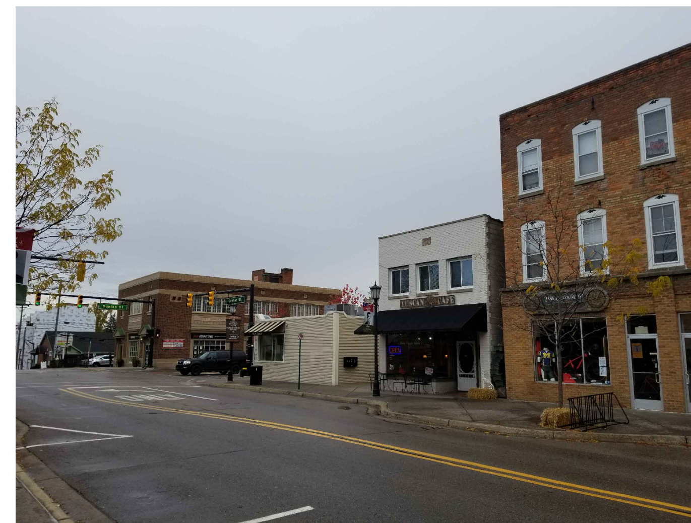
EXISTING LOOKING NORTHEAST
