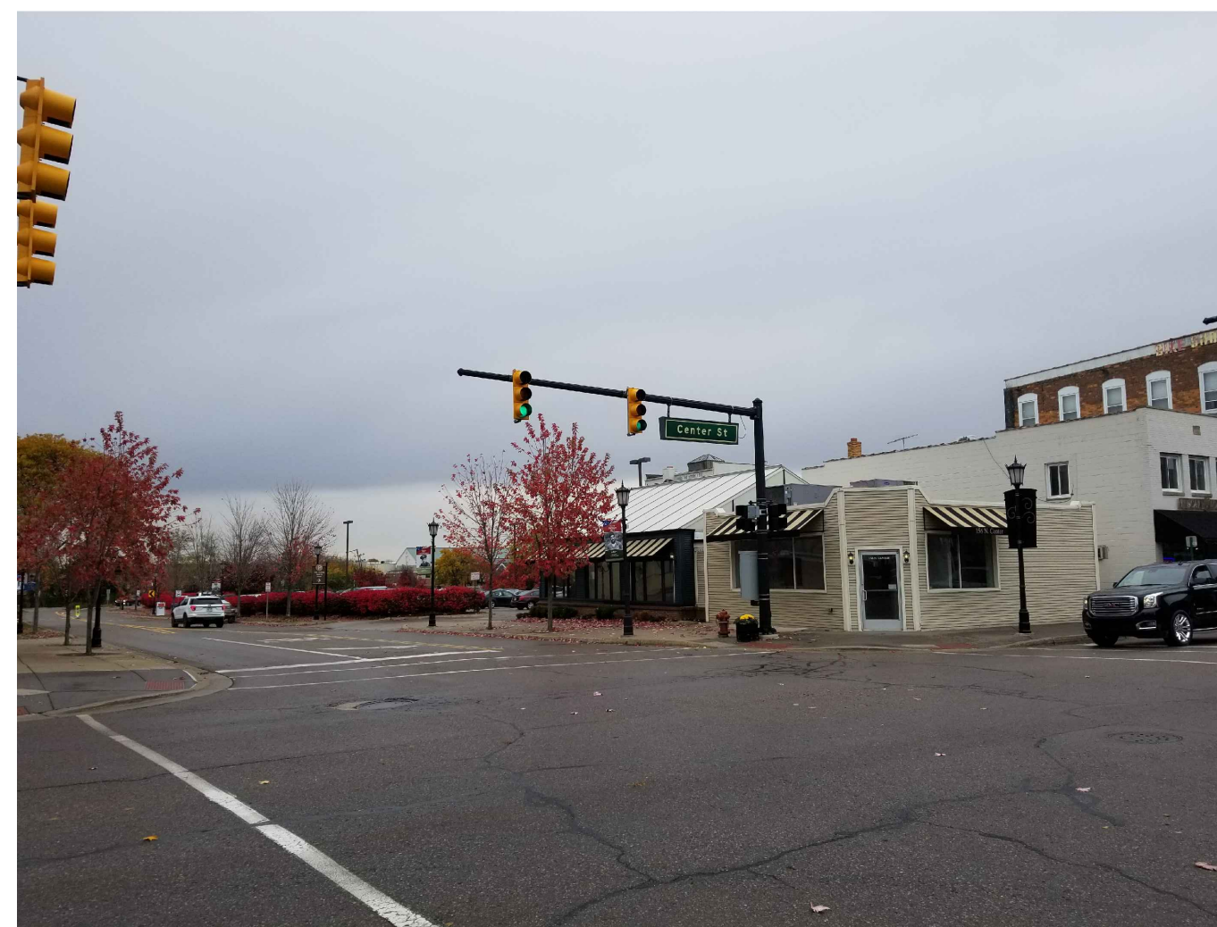
EXISTING LOOKING SOUTHEAST
