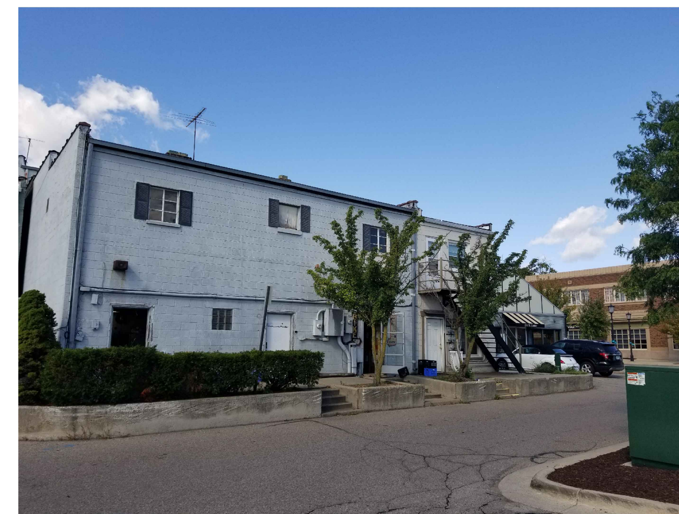
EXISTING LOOKING NORTHWEST
