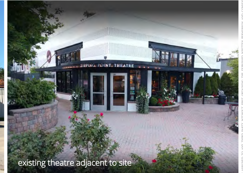
existing building adjacent to site
